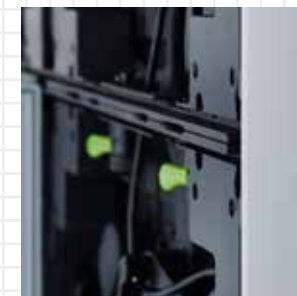
▲ The cabinets are aligned by magnets and two manual connectors to create a sturdy join.
